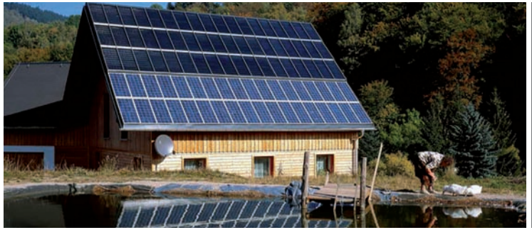
Solar thermal collectors with TiNOX absorbers deliver free, carbon-neutral and reliable heat.
